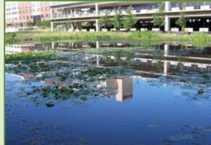
Completed wetland and new hotel at Edgewater Wetland Park in Coralville.
