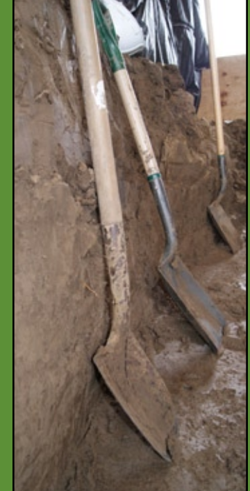
Shovels resting on trench wall at the Palace Site in Des Moines.
