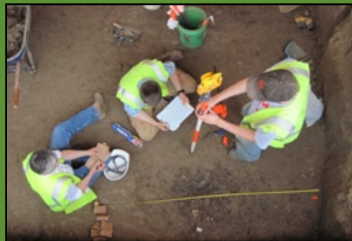
Mapping features at the Palace Site in Des Moines using a total station.
